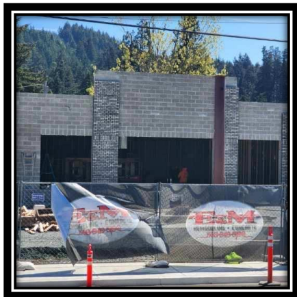
New Service Station on S. 6 th Street
