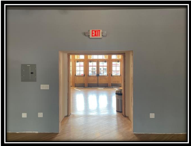
Cottage Grove Armory Drill Hall Entry Remodel
