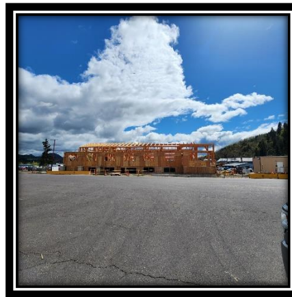
New Administration Building at Starfire Lumber
