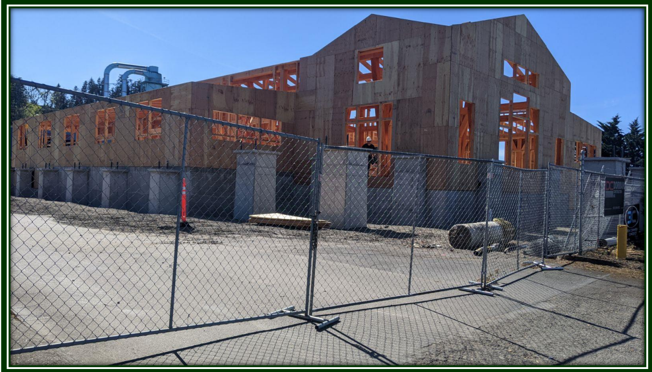
New 18,000 SF office building for Starfire Lumber
