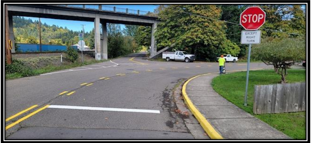
Douglas and Ostrander Street Intersection Restriping and Stop Sign Installation
