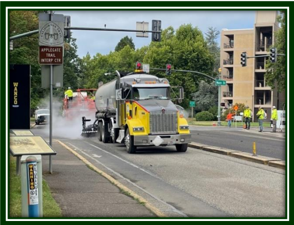
Application of sealer over the new chip seal
