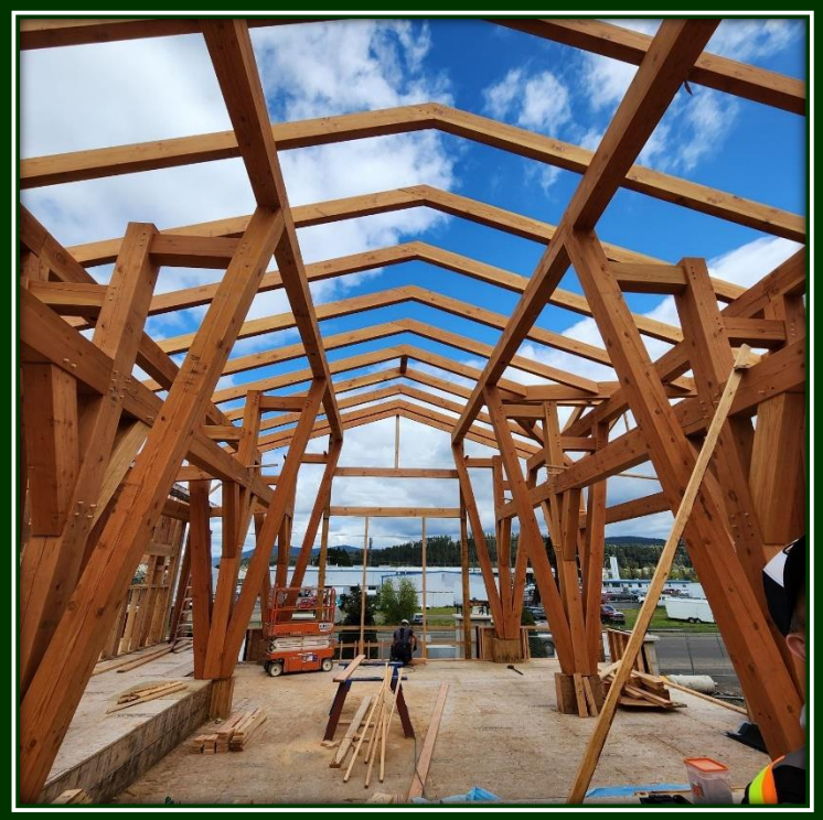
Timber framing for Starfire Lumber’s new office building
