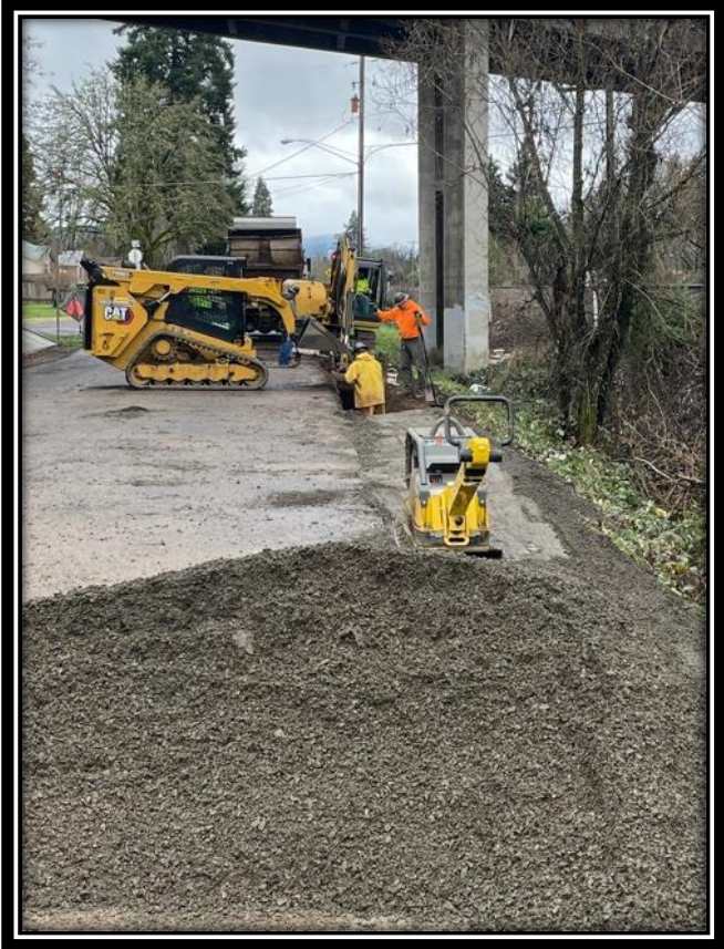
Installation of new 12" effluent line in Douglas Street
