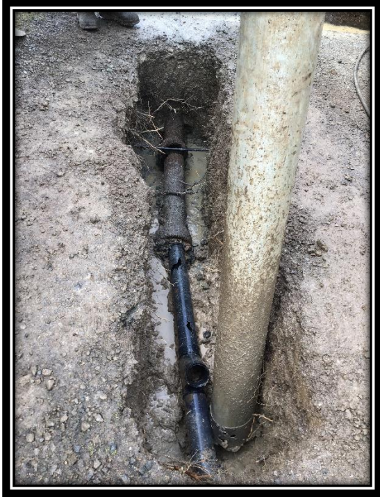
Lateral Sewer Line Repair on South S Street
