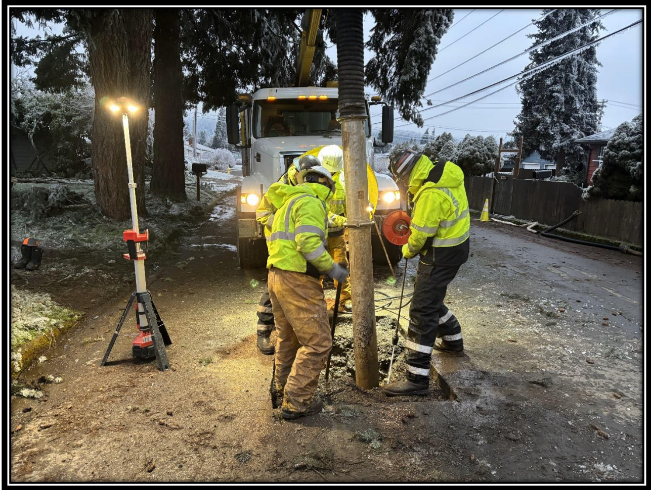
Water Main Line Repair during 2024 Ice Storm
