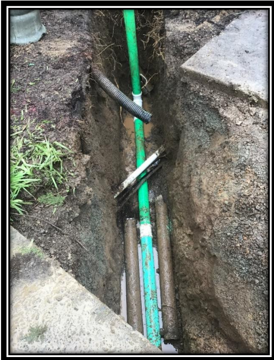
Lateral Sewer Line Repair on T Court
