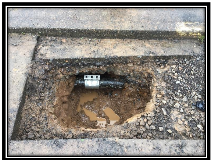
Water Mainline Repair on South 8 th Street
