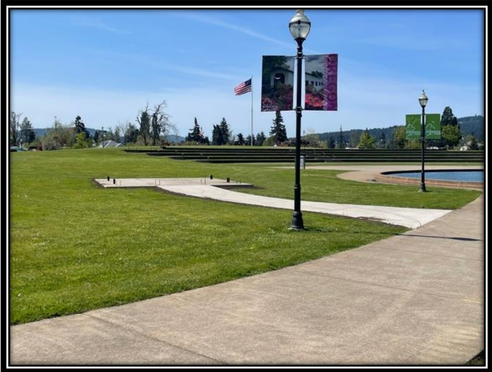
Foundation for the new Picnic Pavilion/Outdoor Classroom
