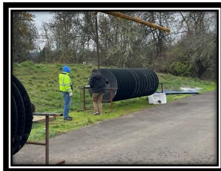
Water Reclamation Plant New Orbital Shaft
