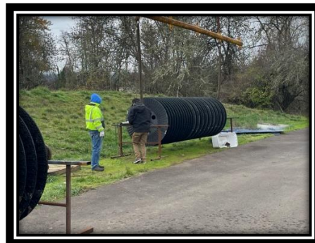
Water Reclamation Plant New Orbital Shaft
