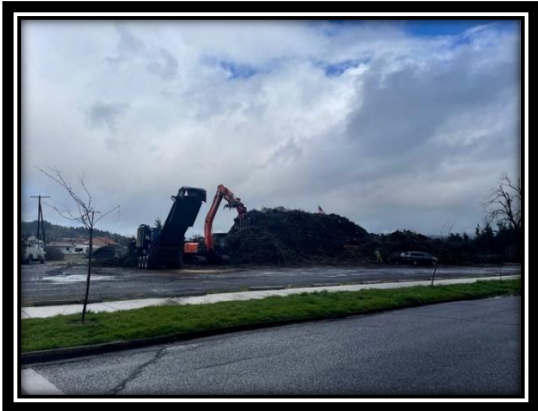
Brush Grinding of 2024 Ice Storm Debris
