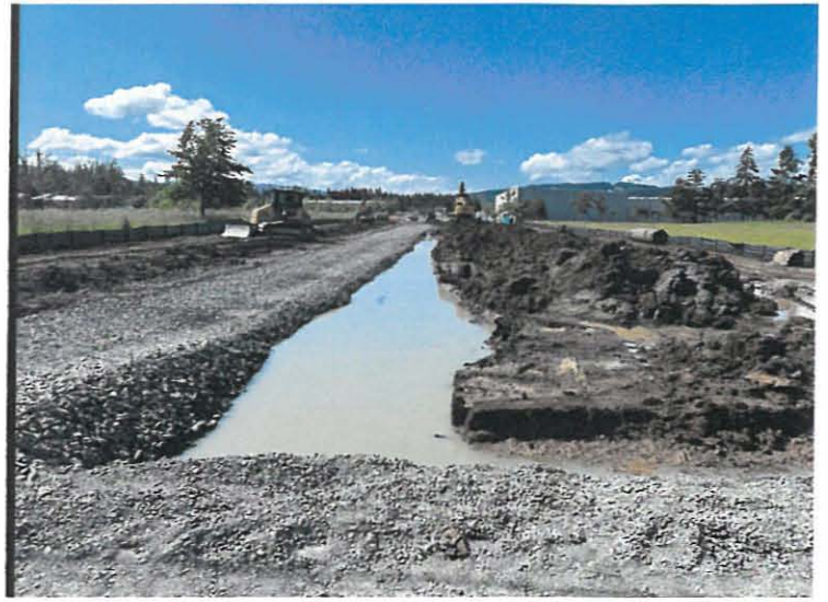
North Subgrade Area
