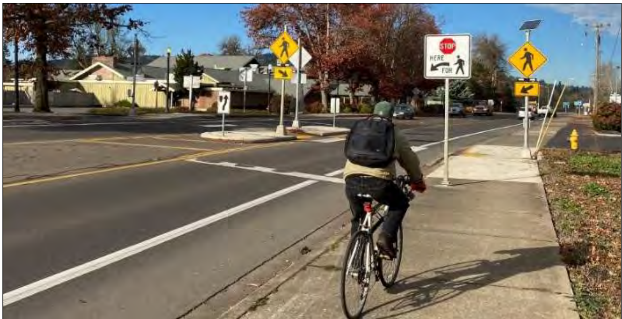
Figure 3-26. Marked Crosswalk with RRFB and Median Refuge on Row River Road
