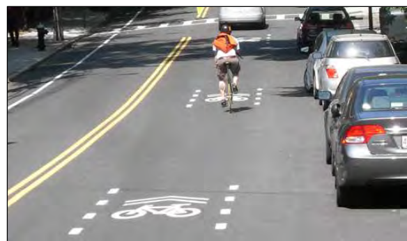
Figure 2-10. Typical Enhanced Shared Roadway
