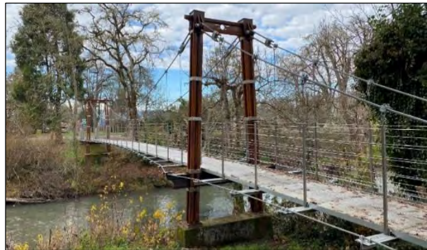
Figure 3-12. Swinging Bridge at Madison Avenue
