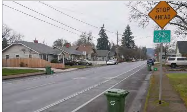
Figure 3-13. Typical Striped Bike Lane and Supplemental Signage
