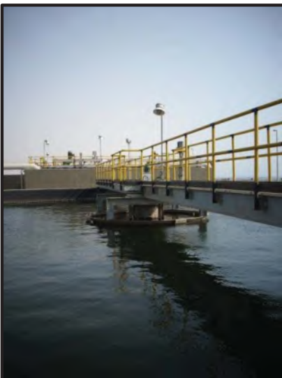
35M CLARIFIER – SAUDI ARABIA
